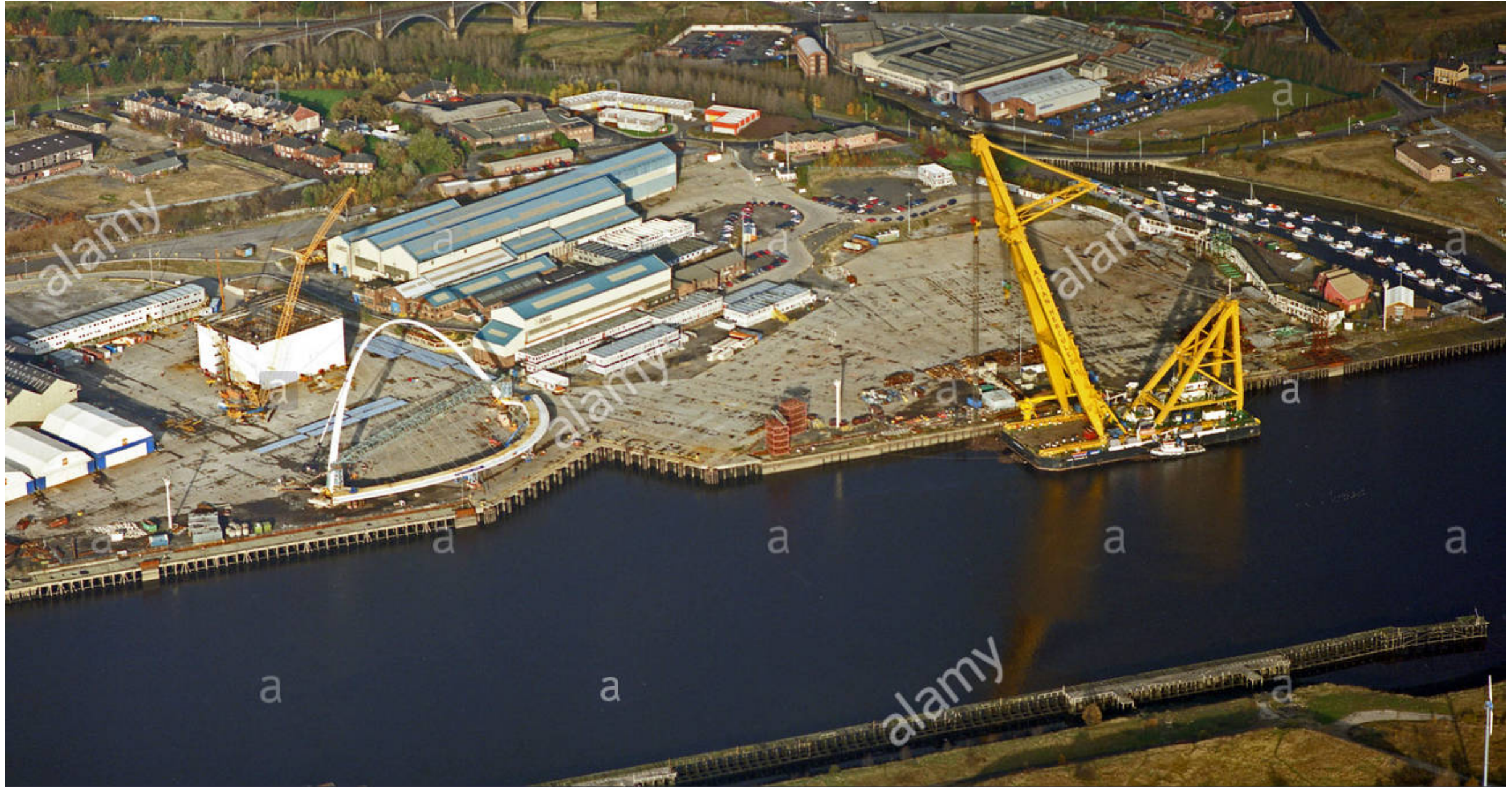
Fabrication of the Gateshead Millennium Bridge takes place offsite: Bridge completely prefabricated and shipped to site.
